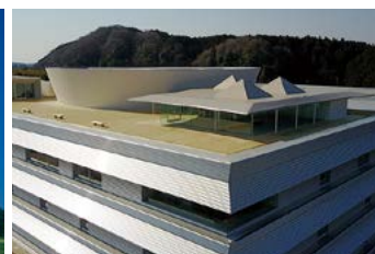
Building exterior showing Sigma environmental control panels
