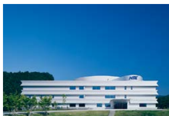
RD1 headquarters building
