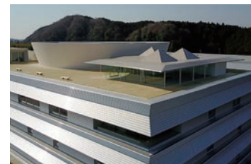
Building exterior showing Sigma environmental control panels
