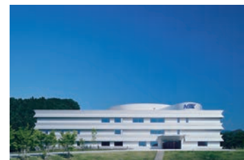
RD1 headquarters building
