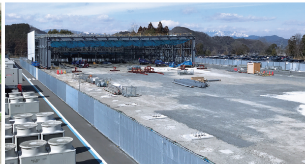
▲ A1+ construction site
